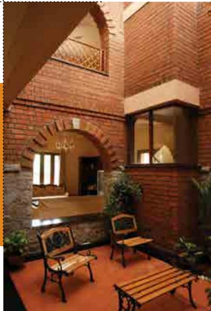
ambience. Being mud walls, they also eliminate the possibility of adding another floor. The roof too is light, being tiled, further suiting the hot weather conditions", adds Khalid. The mud walls essentially are constructed from a mixture of mud, sand and sawdust and shaped to the required form.
