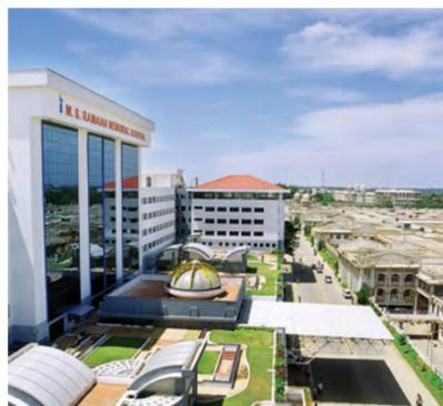
The design is oriented to bring in plenty of natural light and ventilation through presence of internal courtyards and skylights throughout the building. The 7-storied block is North-South oriented with the shorter sides of the building facing East-West. The northern façade is covered fully with glazing that brings flooding natural light into the internal spaces. The
