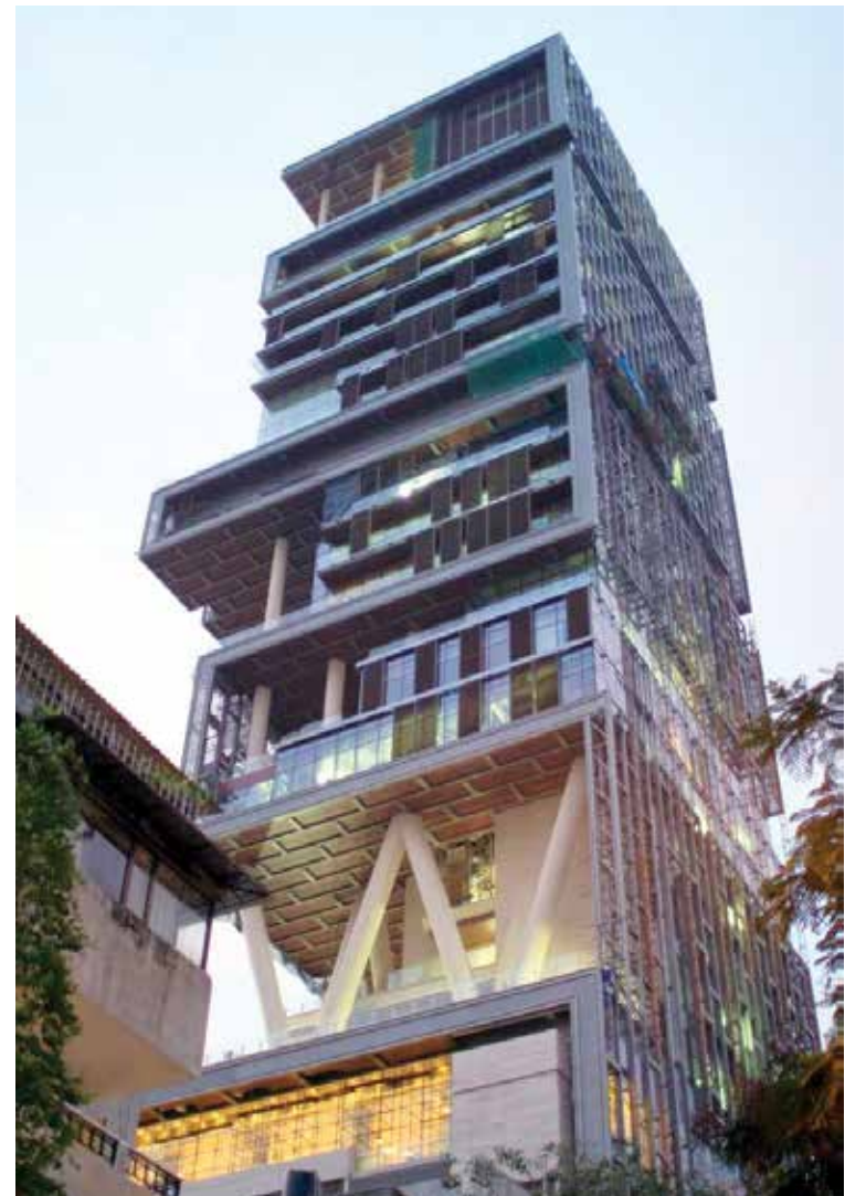
Antilla Residential Towers, Mumbai; Source: Wikimedia Commons
