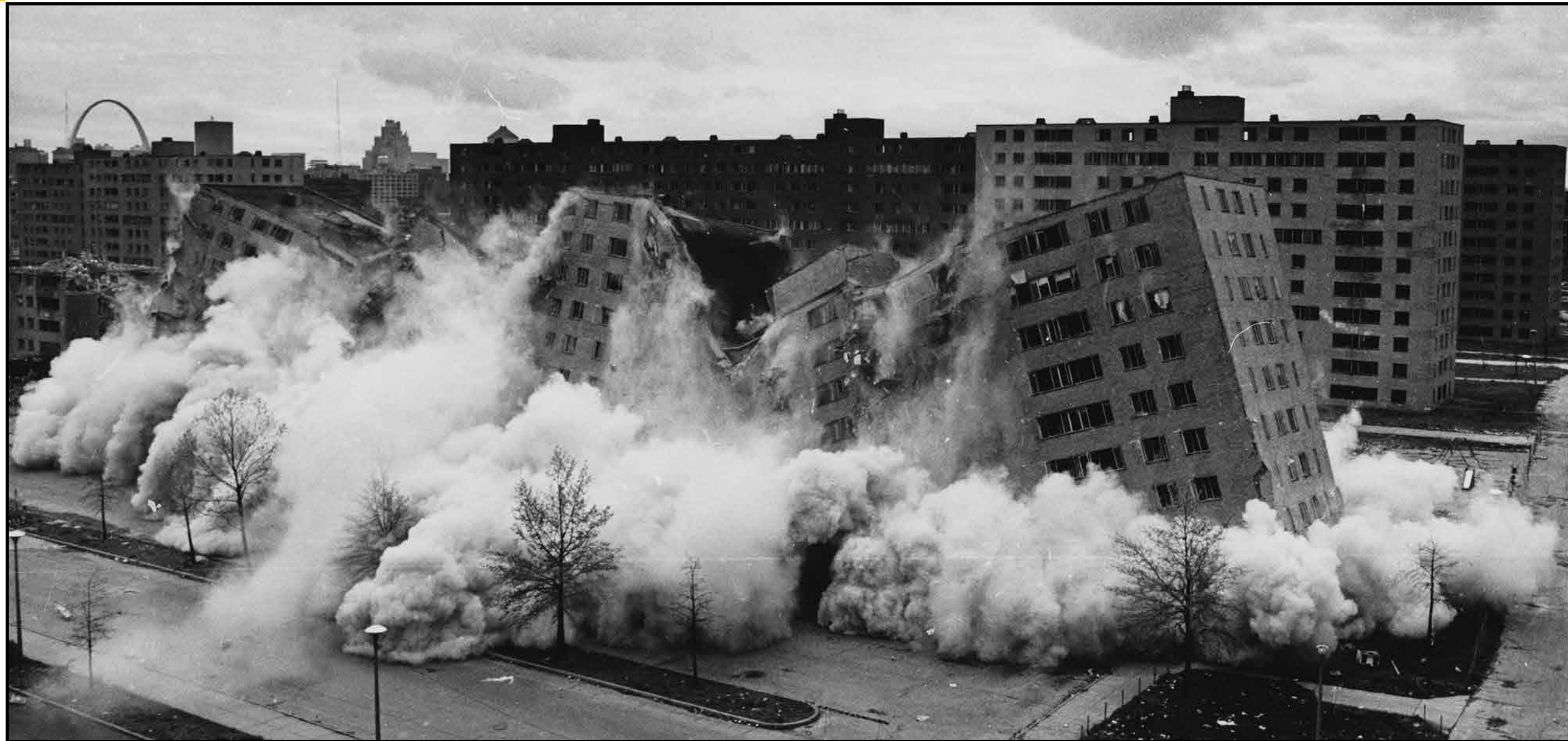
The Pruitt-Igoe complex (demolished as from 1972 to 1976) was composed of 33 buildings of 11 stories each, located on 57 acres[5] of the Near North Side of St. Louis, Missouri. Source: Wikimedia Commons
