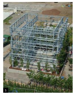
After testing this construction system with over 10 different species of trees, it was observed unfortunately, that not all trees are suitable for this creative method of construction. Trees with thin, flaky barks – that are flexible and robust are best suited for this method. In the Indian context, ficus variants, chinar tree and the Indian banyan tree would be ideal choices.
