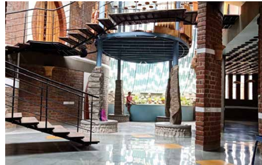
MS pipes support the floating library over the double-height living space.
