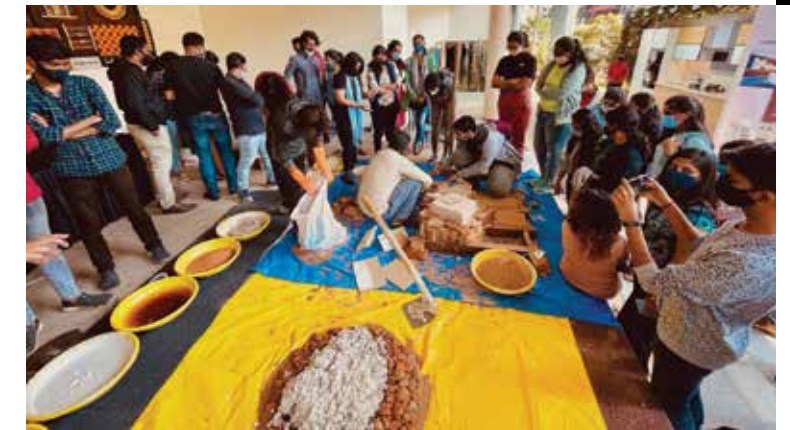
Madras Terrace Roofing Demonstration by INTACH.
