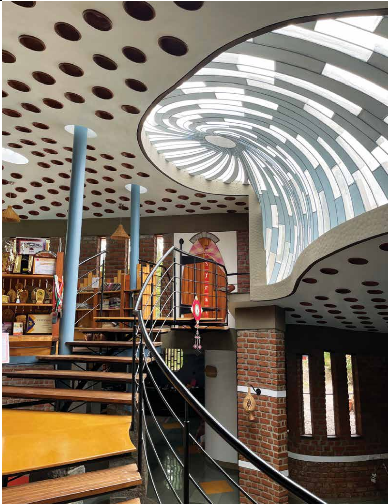
Filler slab roof with the central skylight..
