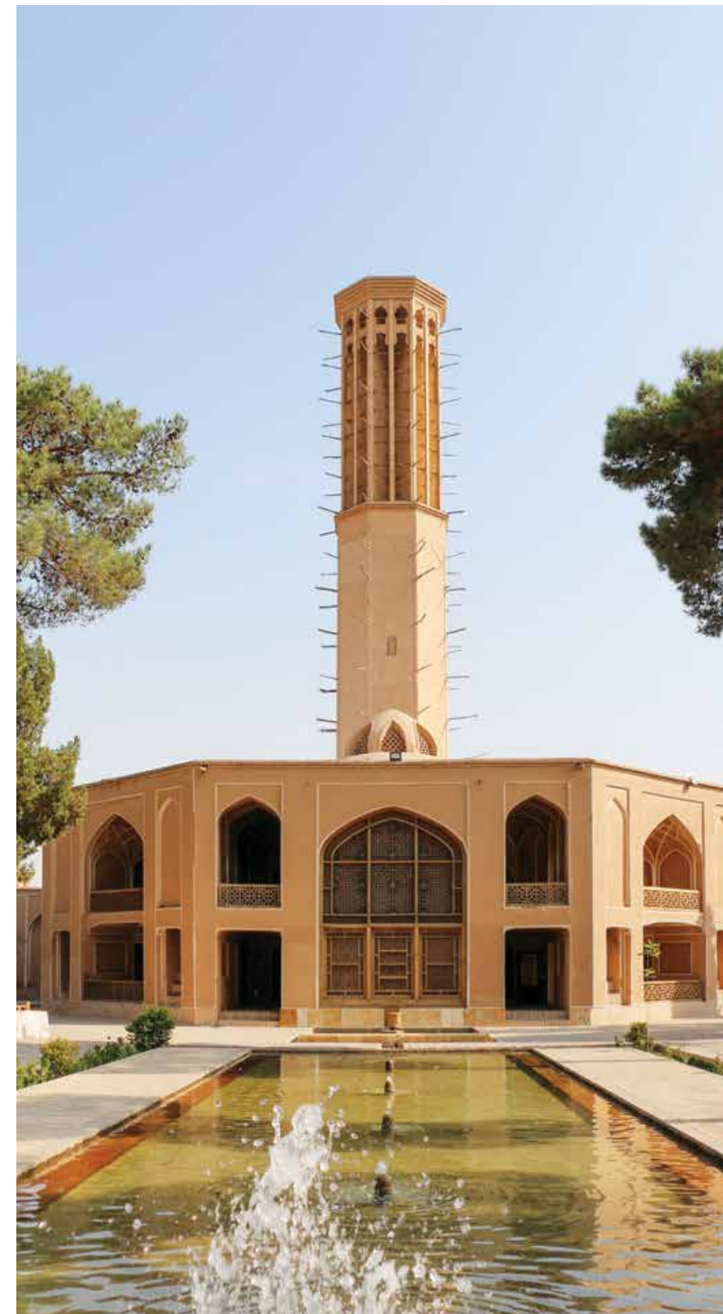
Above: Pavilion in the Dolat Abad Garden with wind catcher, Yazd, Iran. Source: Wikicommons
