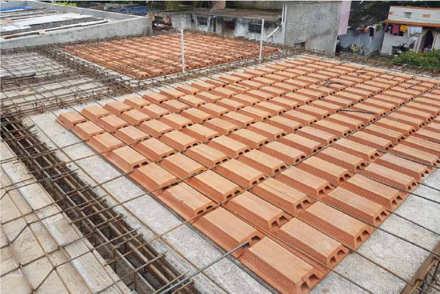
The roof layered with terracotta filler slabs.
