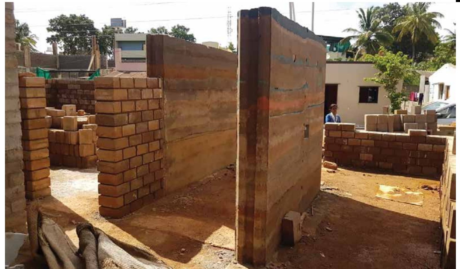
The earthen walls under construction.
