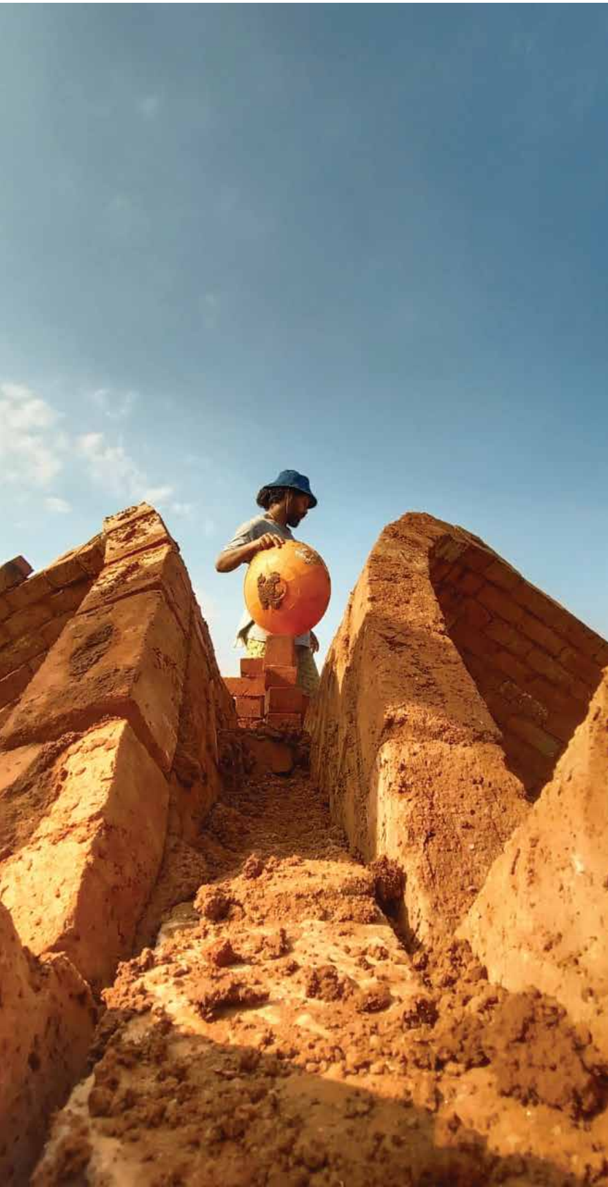
Brick Vault under construction.
