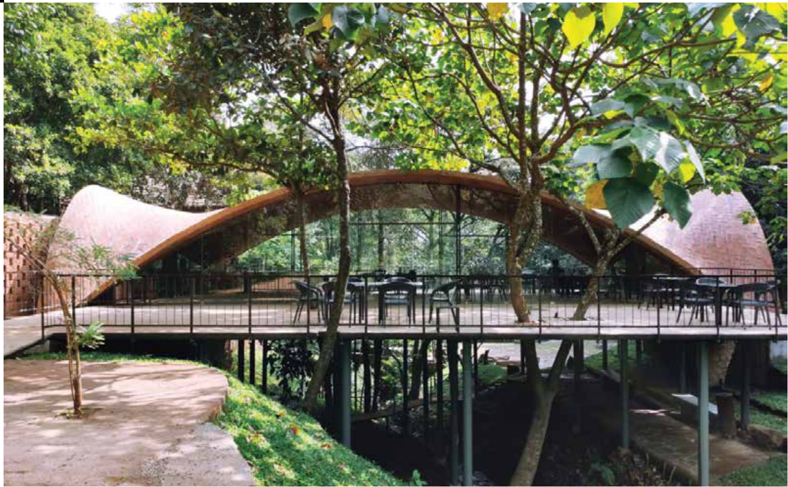
The stone floor built over the valley, the MS pipes blending with the existing trees.
