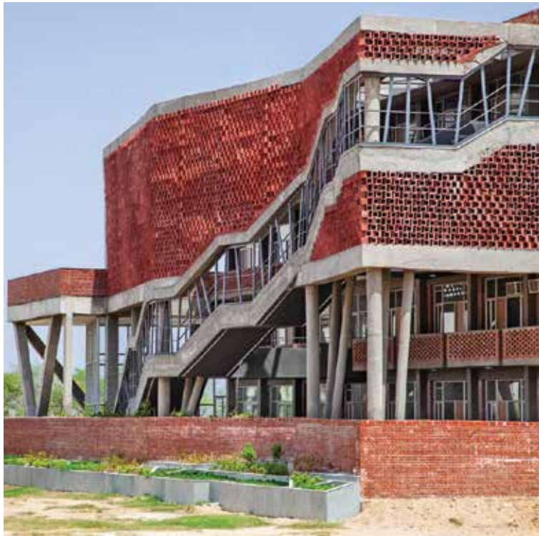
Perforated brick facade enclosing the open to sky courtyard.
