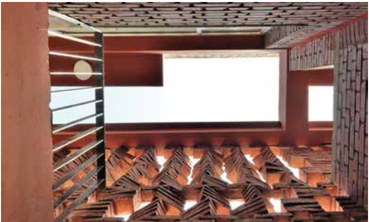
Brick wall structured with rotating bricks.
