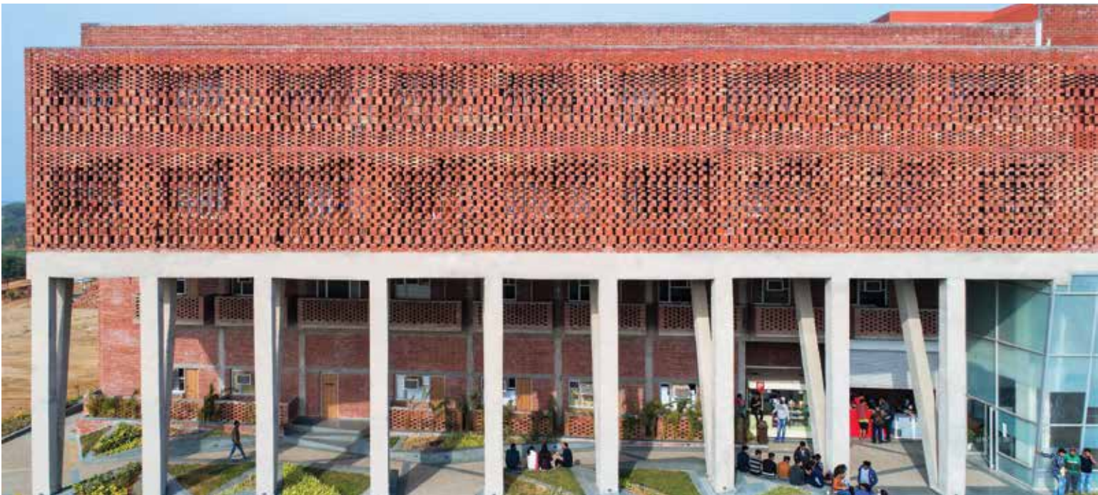
The bricks are angled to lower the direct solar radiation.
