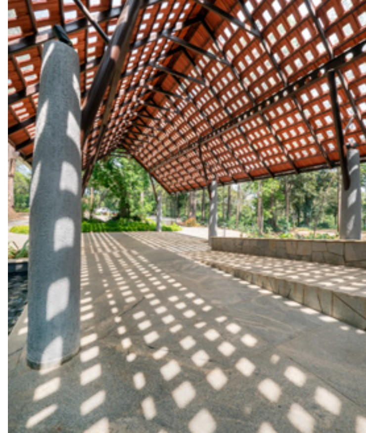
The pavilion gable roof with the glass inset tiles ushers in a mesmerising play of light and shadow
