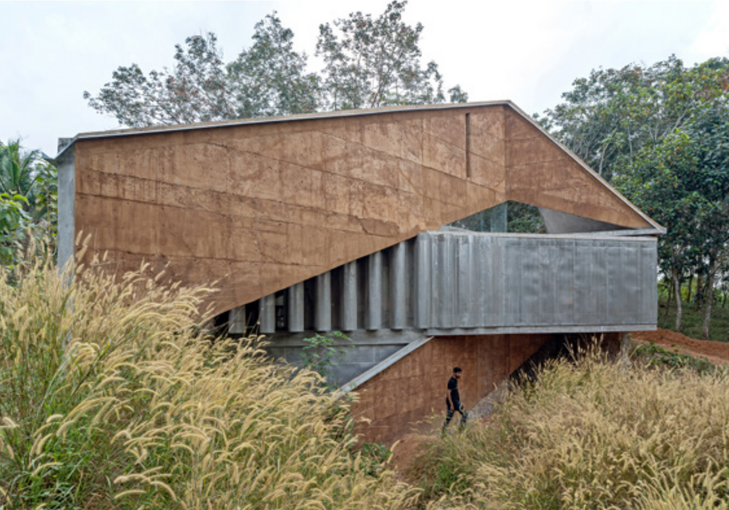
Slanting debris wall designed as a shield against the harsh western sun--Shikara House
