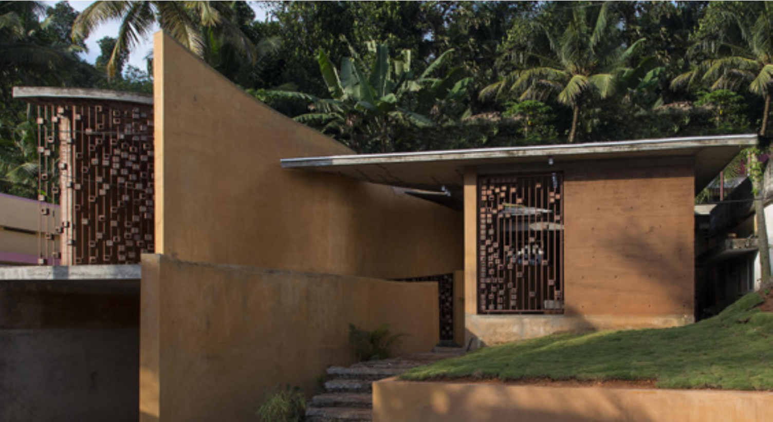
Shuttered debris wall built out of construction debris and earth excavated from the site--Debris House
