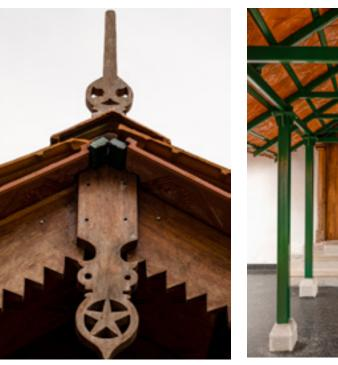
The damaged roof tiles of Maqam Juma Masjid replaced, decayed timber members replaced, multiple layers of paint stripped and replaced with original lime plastering
