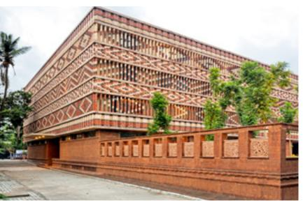
Brick louvered screen serves as a shading device while permitting natural ventilation
