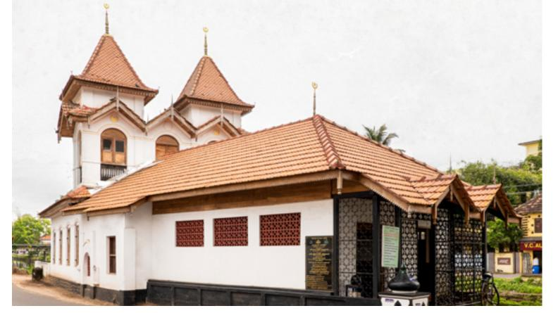
The asbestos roof added later in the Saukar Masjid was removed and replaced with the original form of clay tiles used in the core structure
