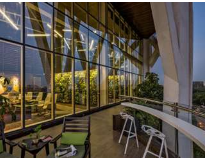
The cylindrical perforated MS envelope of the building not only serves as a sculptural feature but also serves as a shield to the interiors while letting in ample natural light--Nyati Unitree
