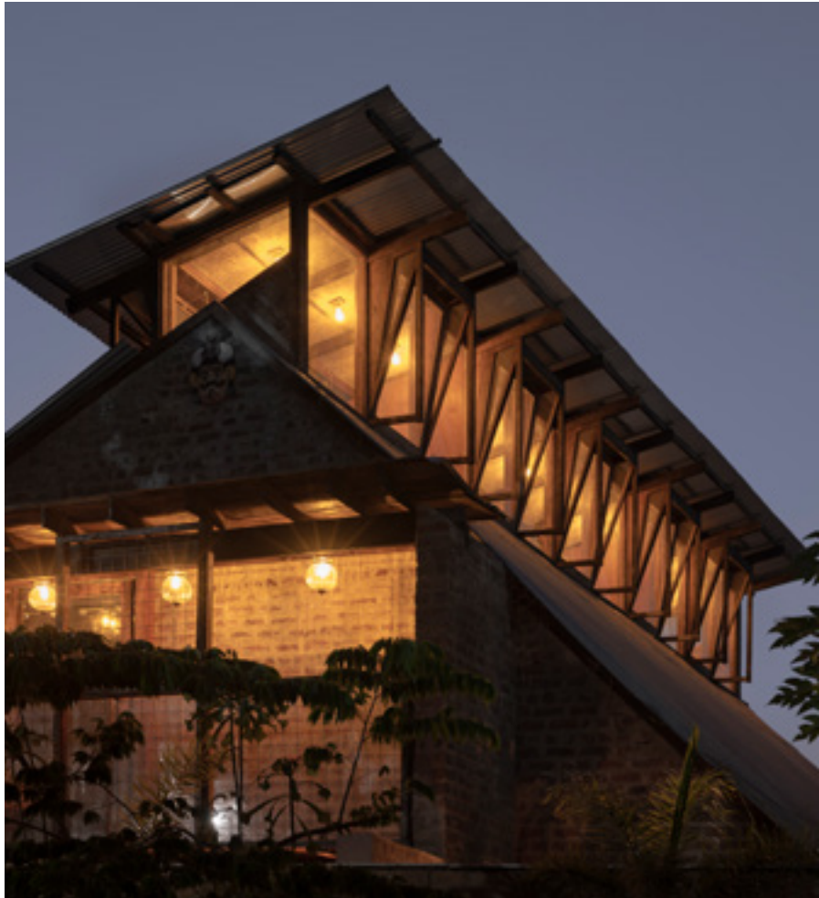
Exterior facade with the brick wall and clerestory windows
