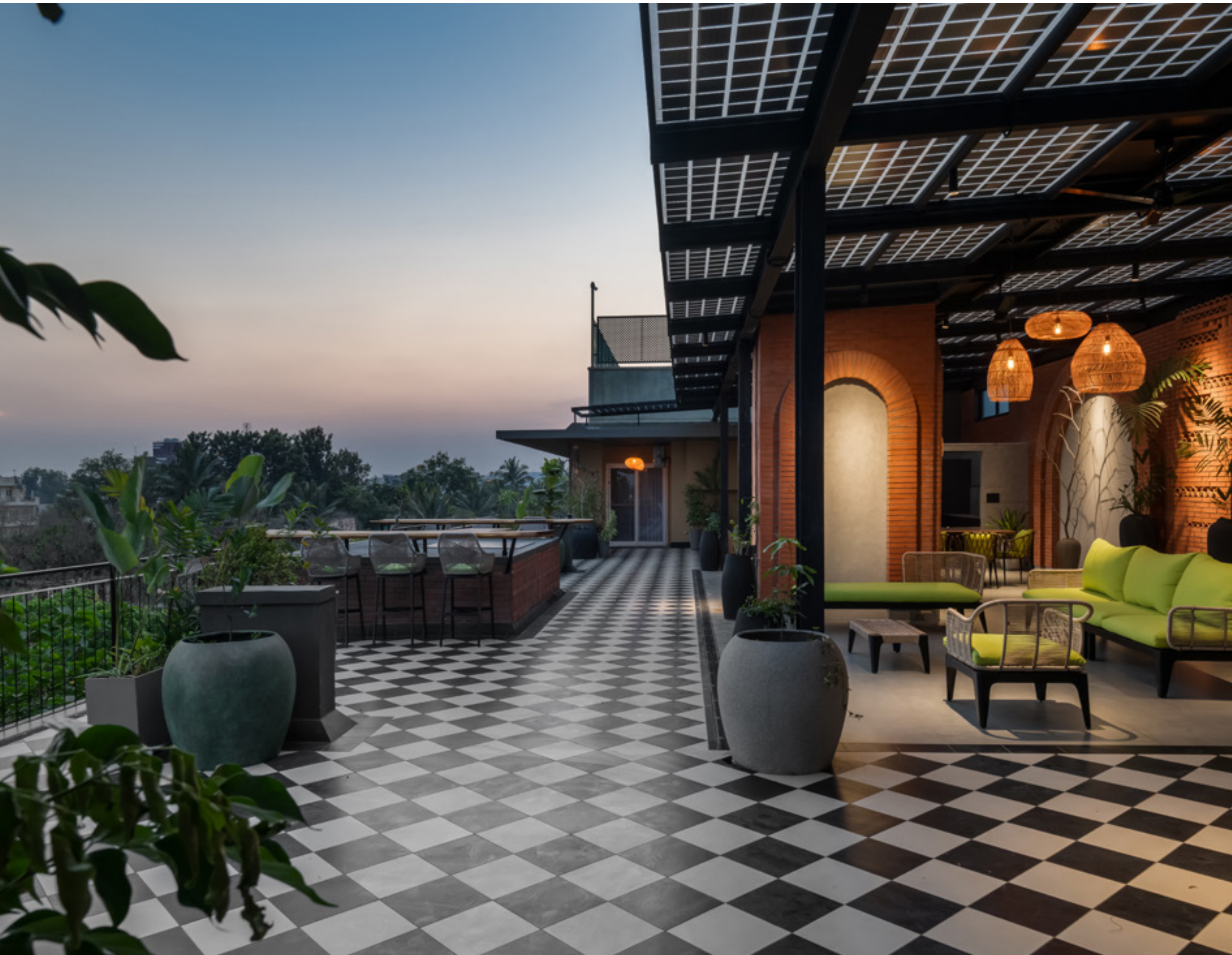
The large terrace is converted into a vibrant open lounge where the solar panels serve as an artistic roof
