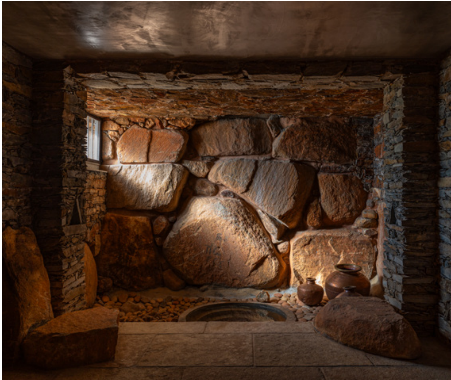
Raw stone boulders form the seating as well as the retaining wall in the basement
