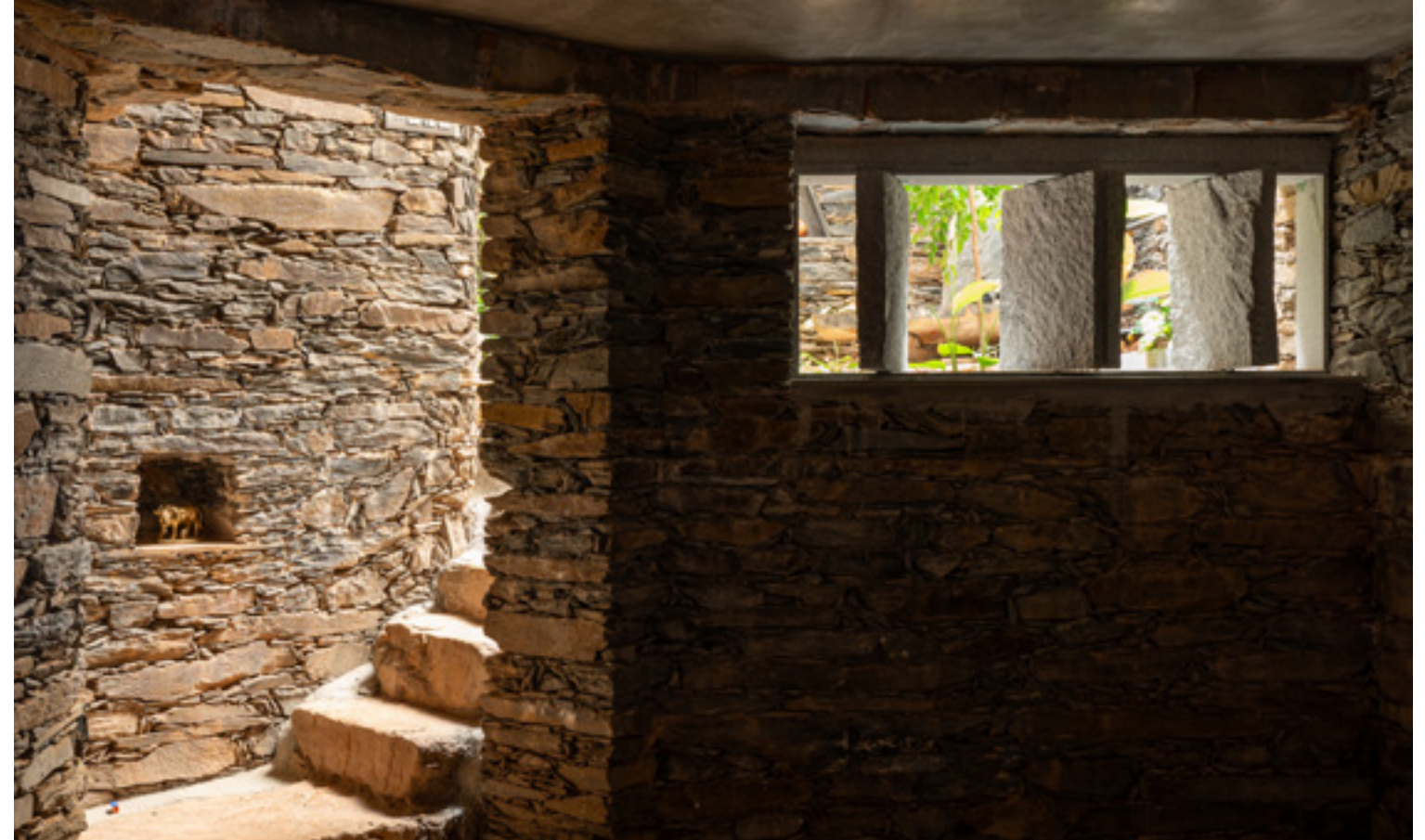
Stone treads, random rubble masonry walls, stone louvered vents mark the basement
