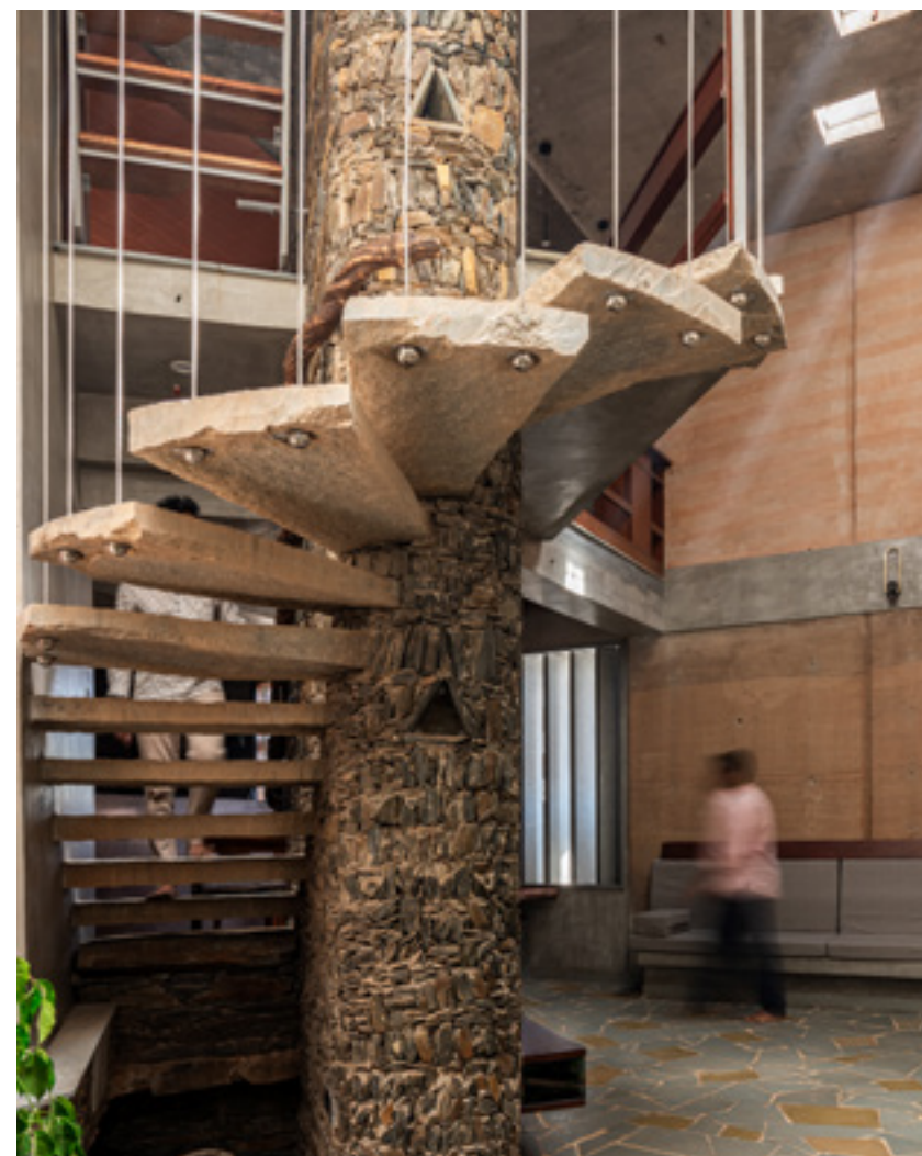
Cantilevered raw stone slabs form an unconventional circular staircase
