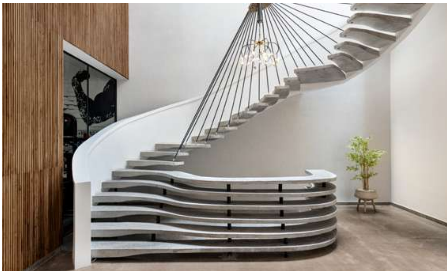
Dramatic installation of cables support the concrete treads while serving as the railing -- Ribbon House
