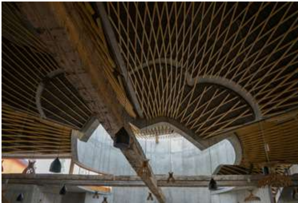
Wooden beams and woven ceiling structure indoors, Source: Unsplash
