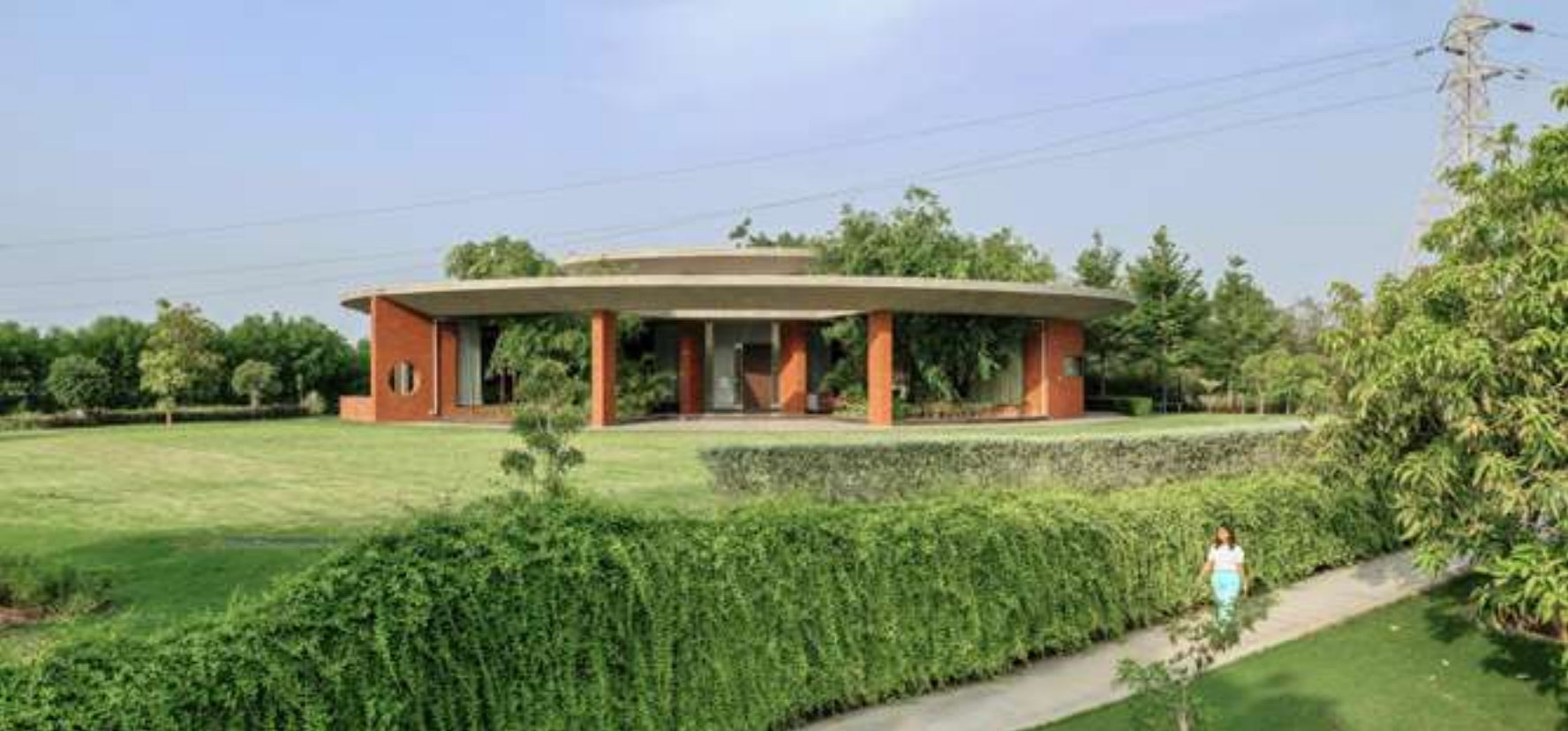
Ring House against the backdrop of lush greens
