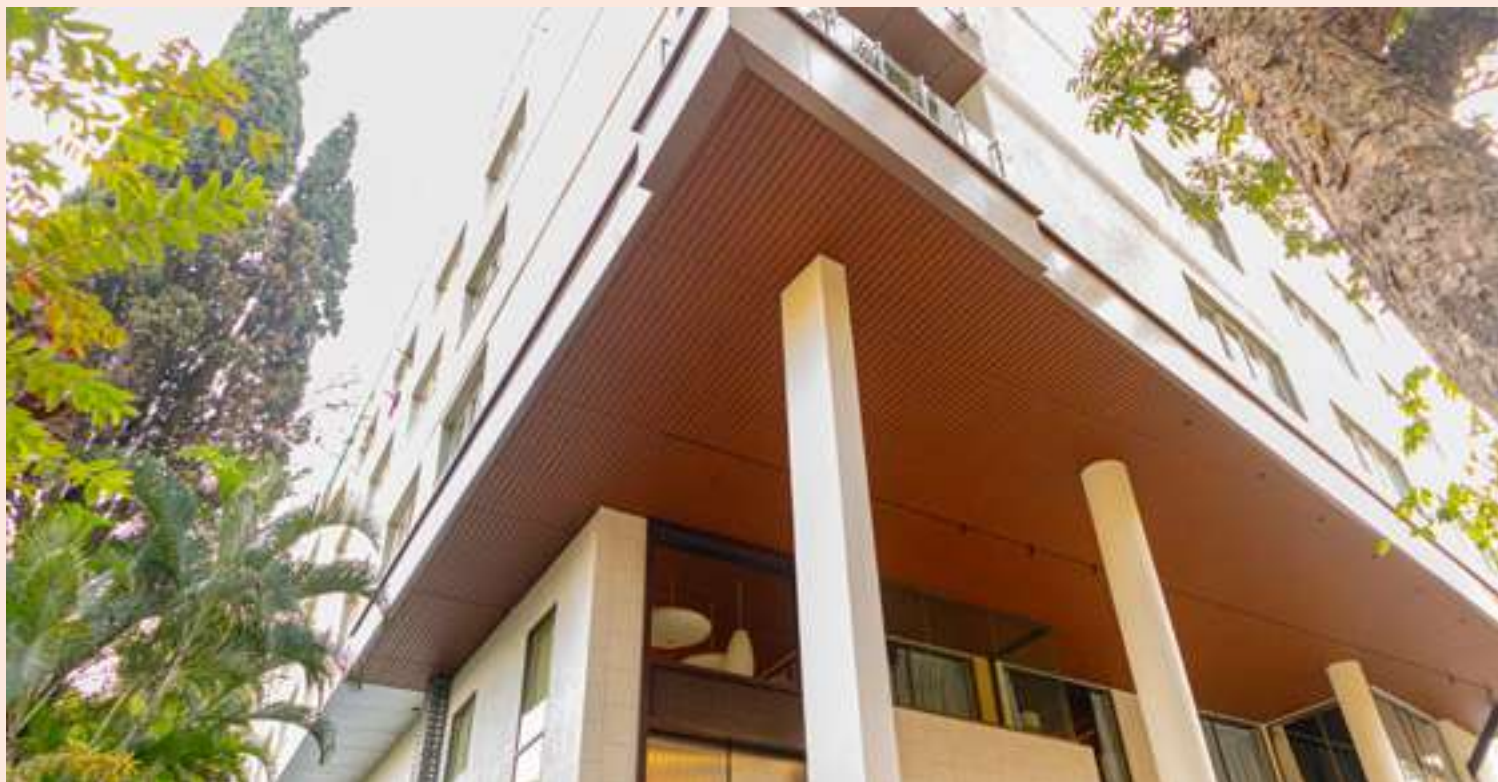
The wood-finish ceiling extends across the sheltered outdoor space, adding warmth to the architecture. The linear panels create a clean and continuous overhead surface.
