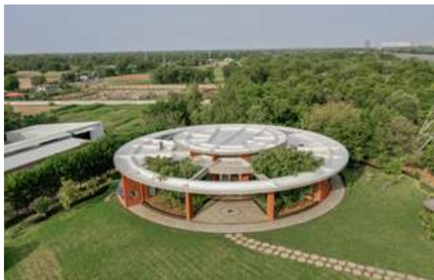
Aerial view of the structure
