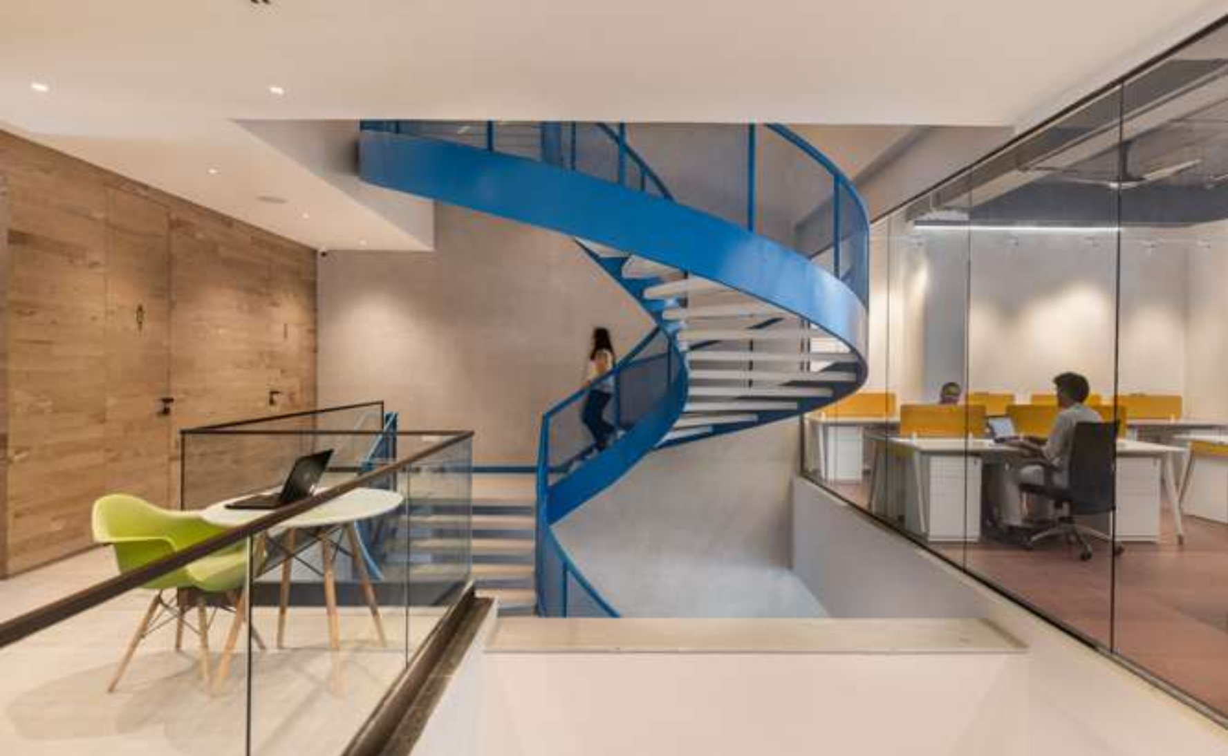
The circular metal staircase crafted from waste metal--Studio Ardete
