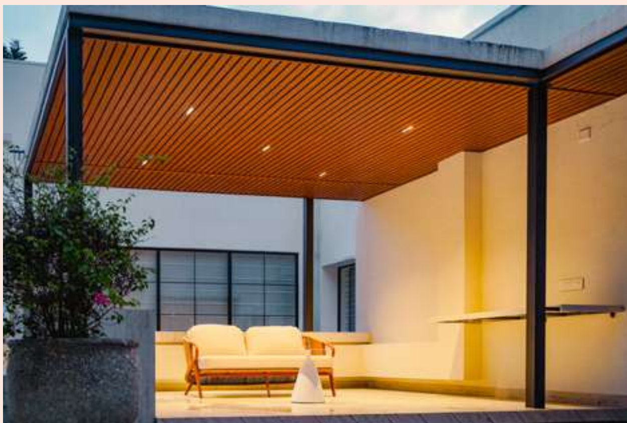
The wood-finish ceiling brings a cohesive visual language to the outdoor seating area. Integrated lighting and linear detailing enhance the sheltered space.
