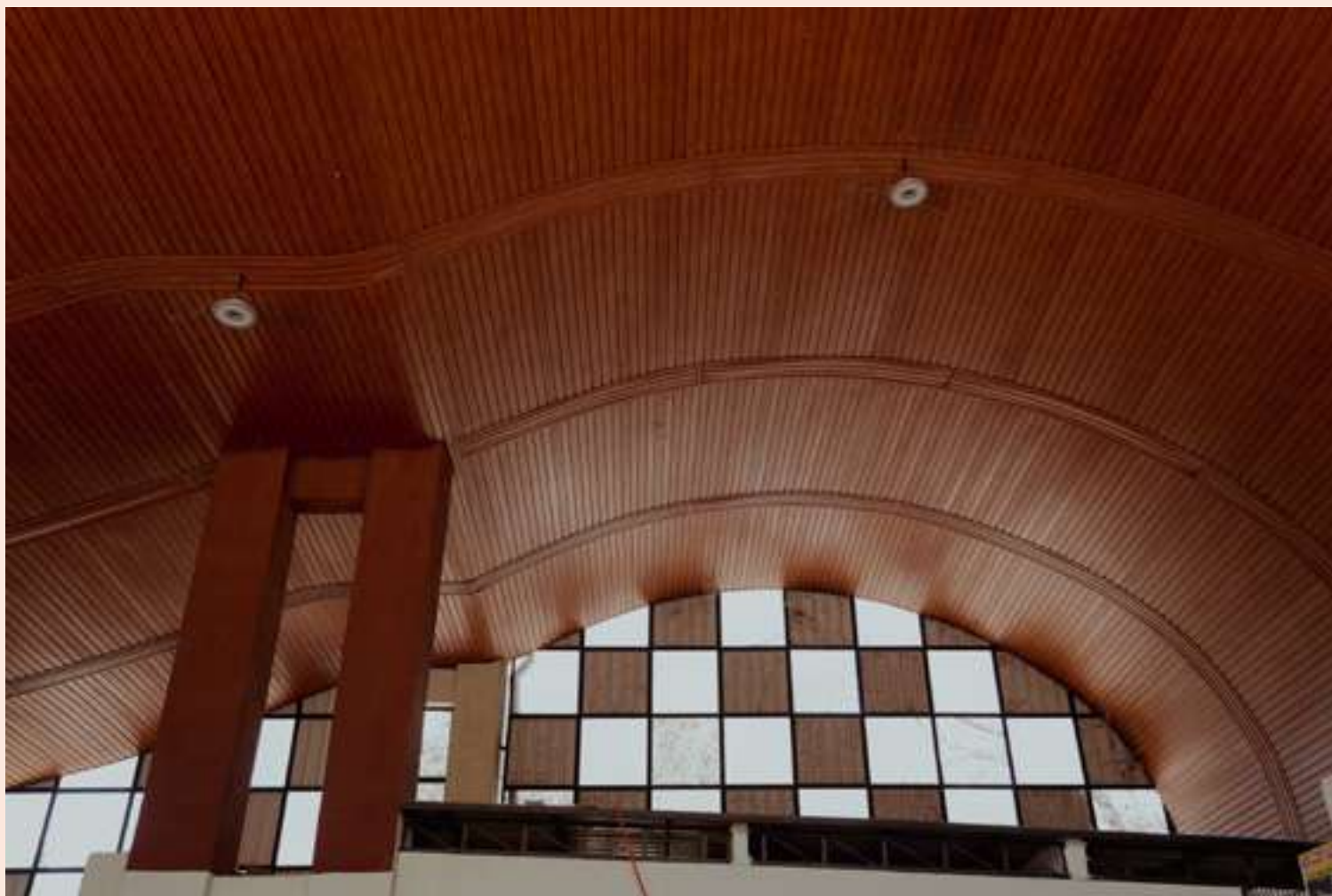
The bus stop's curved ceiling panels flow seamlessly with its sweeping structure, creating a fluid and distinctive overhead form. The wood-inspired finish brings warmth while accentuating its architectural character.
